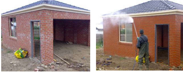
Brick Cleaning - before and after
