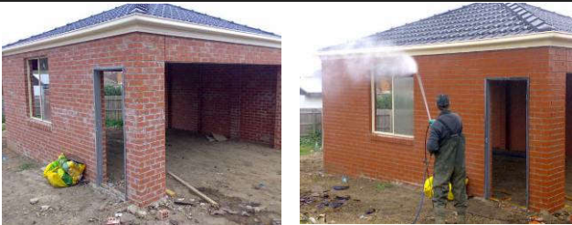
Brick Cleaning - before and after
